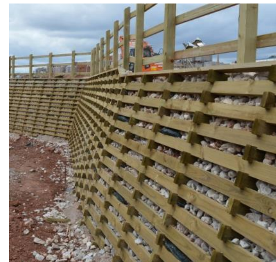
Figure 30 – Typical Permicrib Wall under construction
