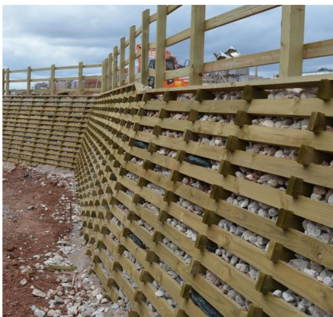
Figure 5 – Typical Permicrib Wall under construction
